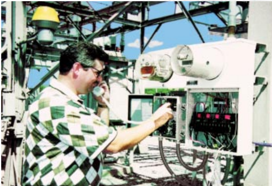
The PQPager gathers and stores data, then automatically pages you when a disturbance occurs. Use the voice-mail-like interface to hear the details from any phone.
